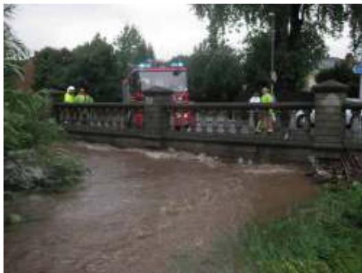
Dogpool Bridge at 17:05BST
